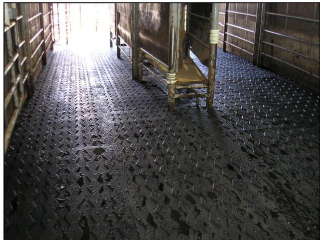
From discussions with RPS it was determined how the SureFoot® Cattle mat could be best utilized to eliminate the maintenance & mess issues the facility currently experienced. A concrete floor was first laid to provide a stable structure to install the RPS SureFoot® Cattle mat.
