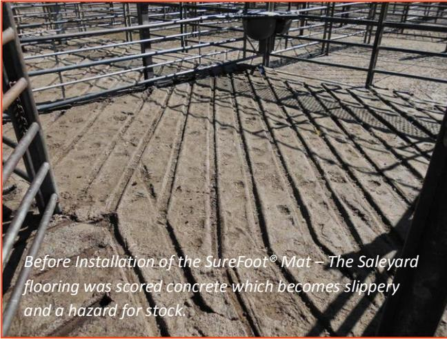
*Before Installation of the SureFoot® Mat – The Saleyard flooring was scored concrete which becomes slippery and a hazard for stock.*
